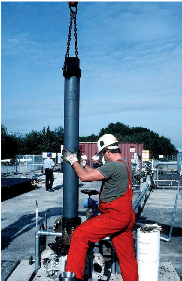
Fig. 41: Pump installation in deep well GB2 (Bruchsal)
