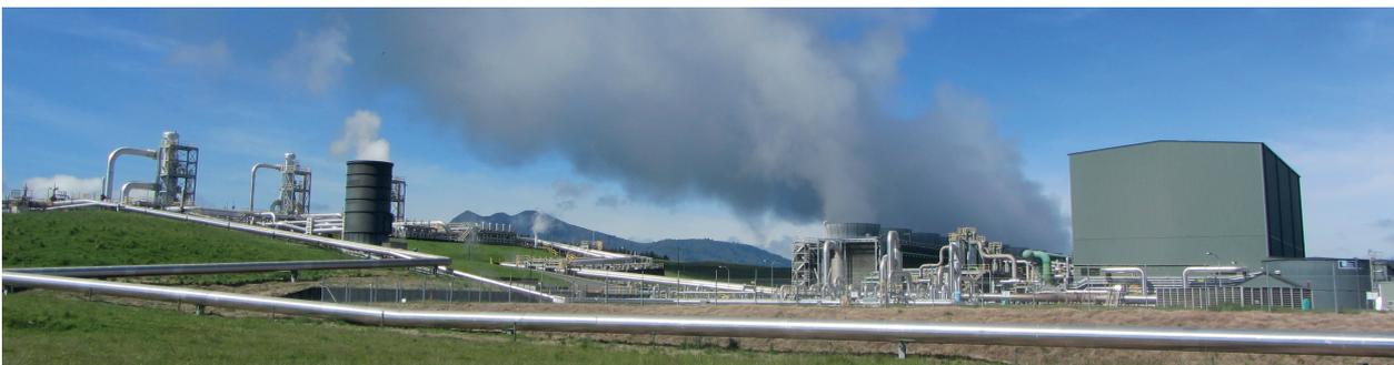
**Figure 4: 140 MW<sub>e</sub> Nga Awa Purua triple flash power station near Taupo, New Zealand.**
